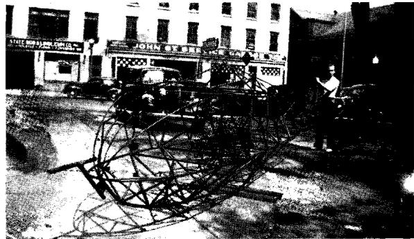
Welded Steel Fuselage Structure.
