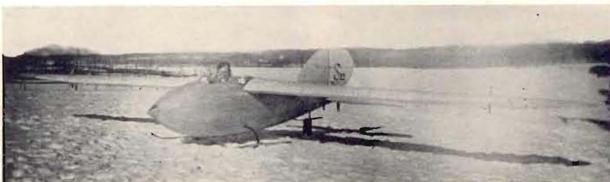
The Gluhareff S-22 (S for Soarer, 22 for the year of construction) with Michael Gluhareff in the open cockpit. It is of special interest in this country because Mr. Gluhareff used the wing airfoil from the S-22 on the U. S. Pratt-Read sailplane which he later designed.
